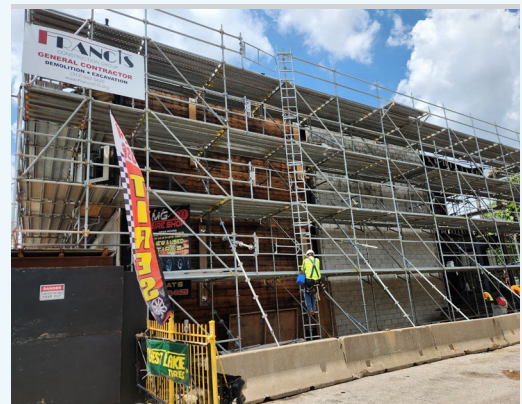
Caption: The E.G. Woode Food Hub at 1022 W. 63rd St, is a $7.1M development currently under construction transforming a 10,500 sq. ft., 113-year-old former mixed-use property into a commercial kitchen, 2 permanent restaurants, a pop-up kitchen for emerging entrepreneurs, and a space for culinary classes and offices.
