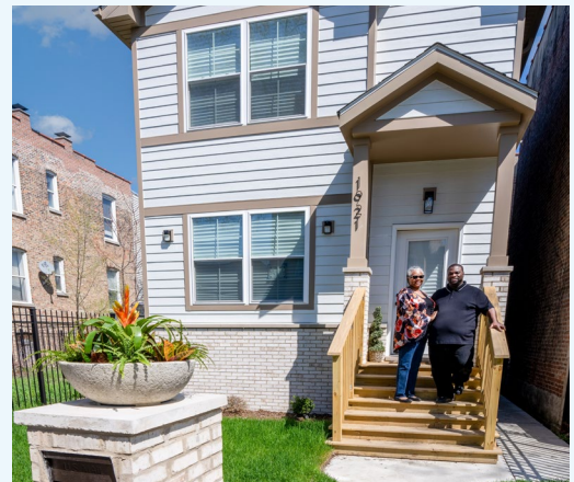
Caption: Reclaiming Chicago is expanding pathways to affordable homeownership across Chicago's South and West Sides.
